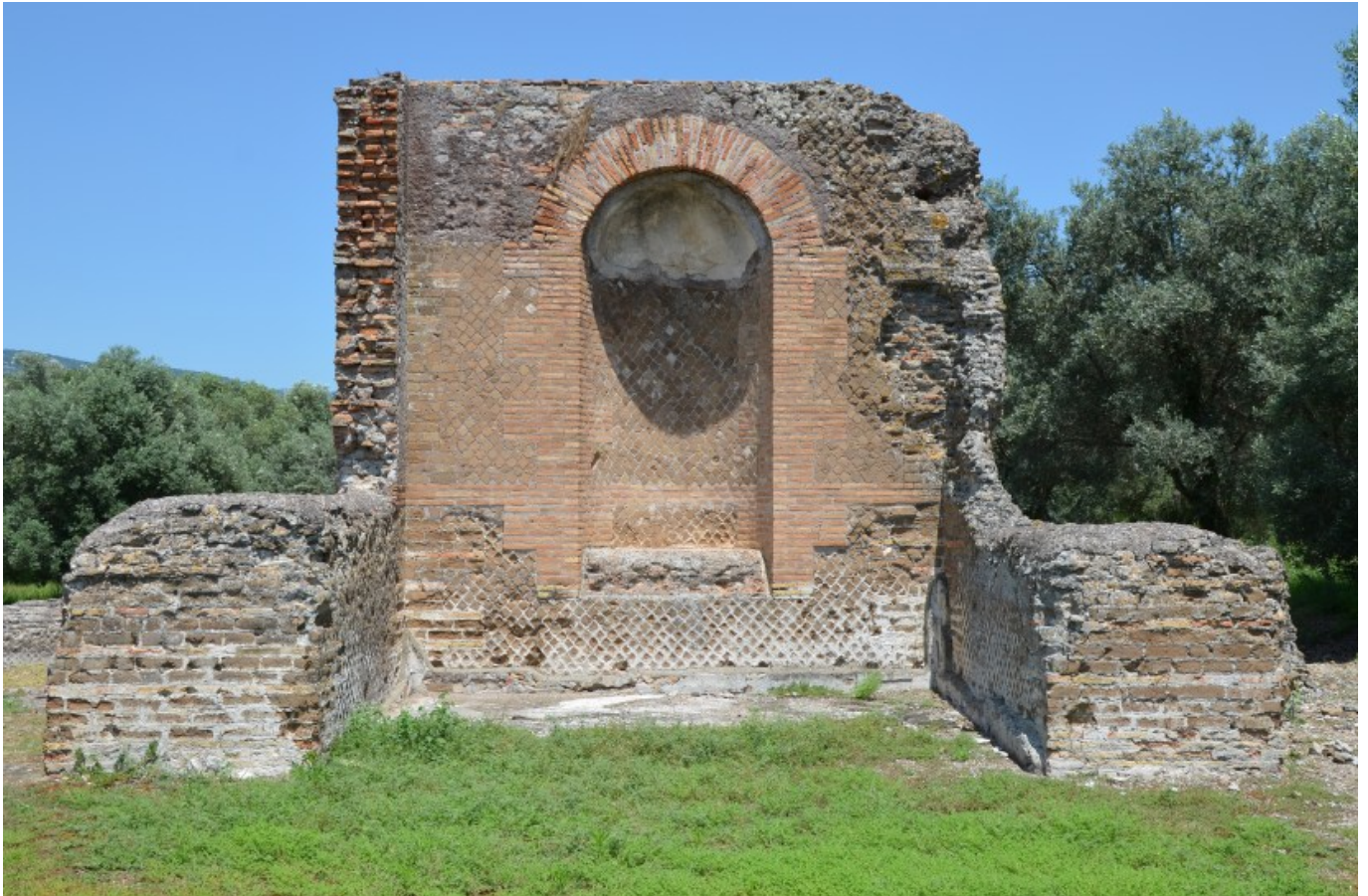
Sala a Tre Navate (Hall of Three Aisles), Imperial Palace complex.
