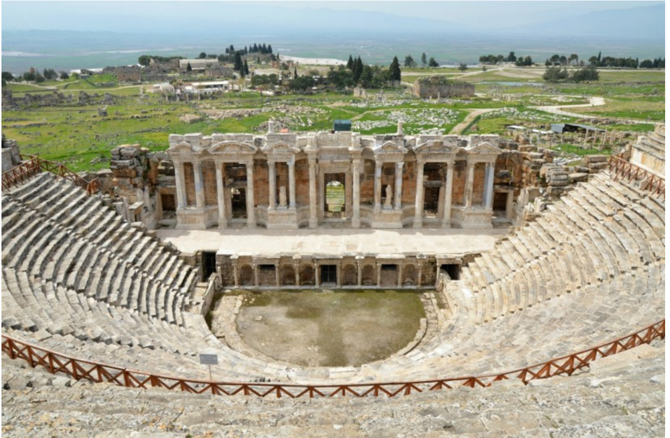
The Roman Theatre of Hierapolis, built in the 2nd century AD under the reign of Hadrian. It has been the object of important restorations between 2004 and 2014.
