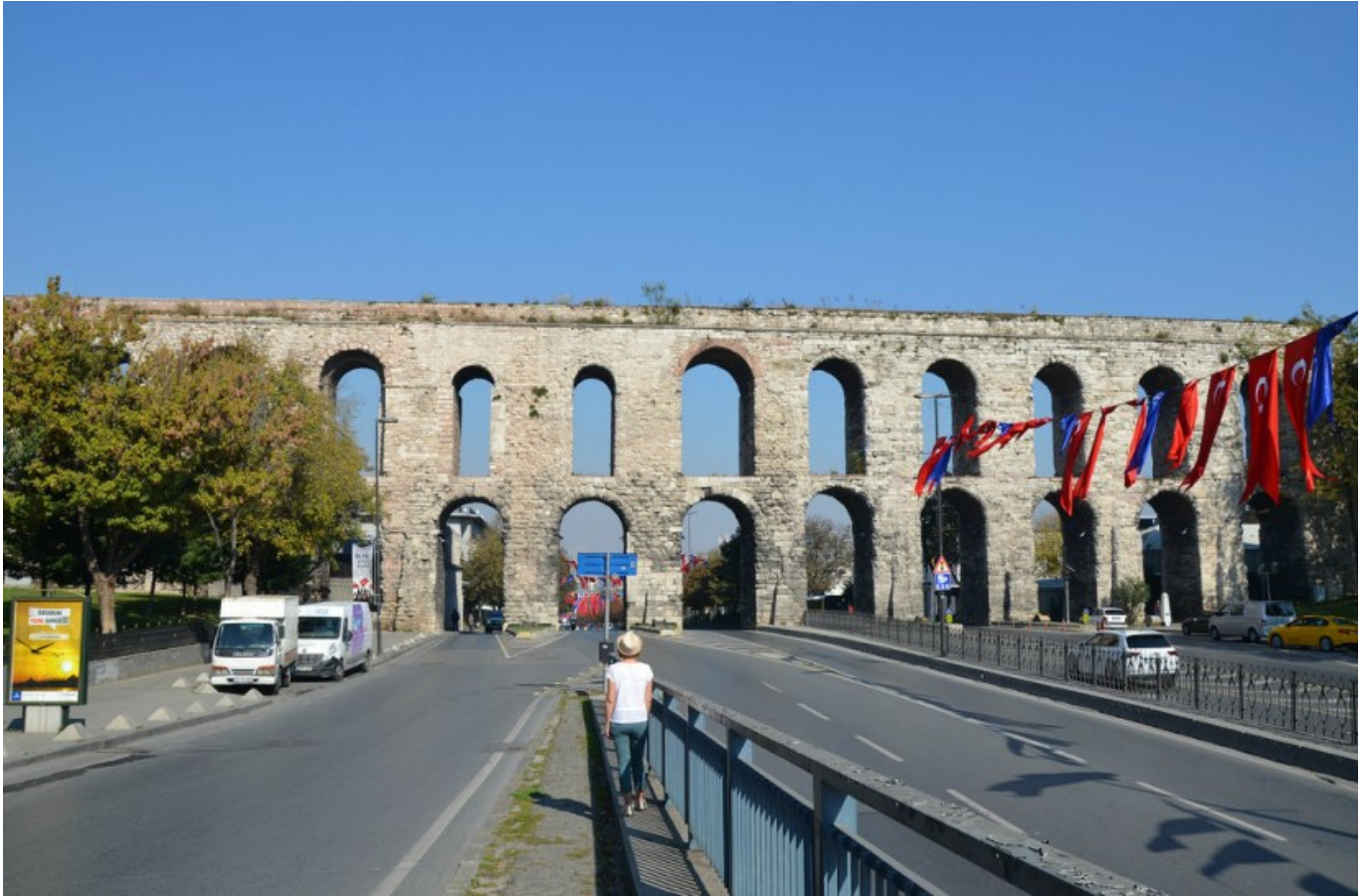
The Valens Aqueduct in Istanbul.
