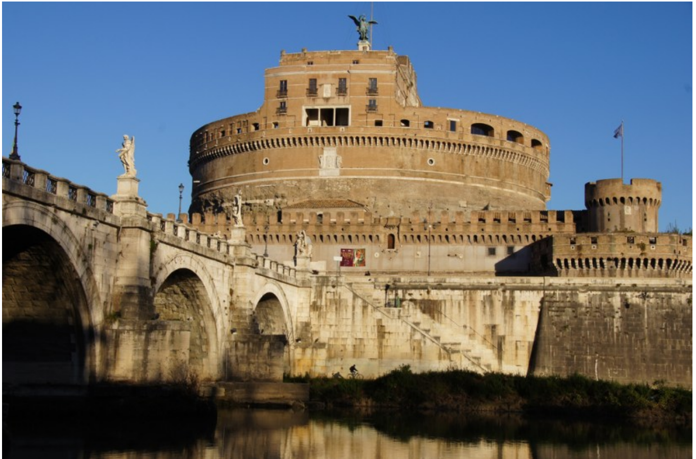
The Mausoleum of Hadrian, completed in AD 139 but since greatly modified to become a Papal fortress known as Castel Sant'Angelo, and the AD 134 Pons Aelius (now the Ponte Sant'Angelo) – Rome, Italy.
