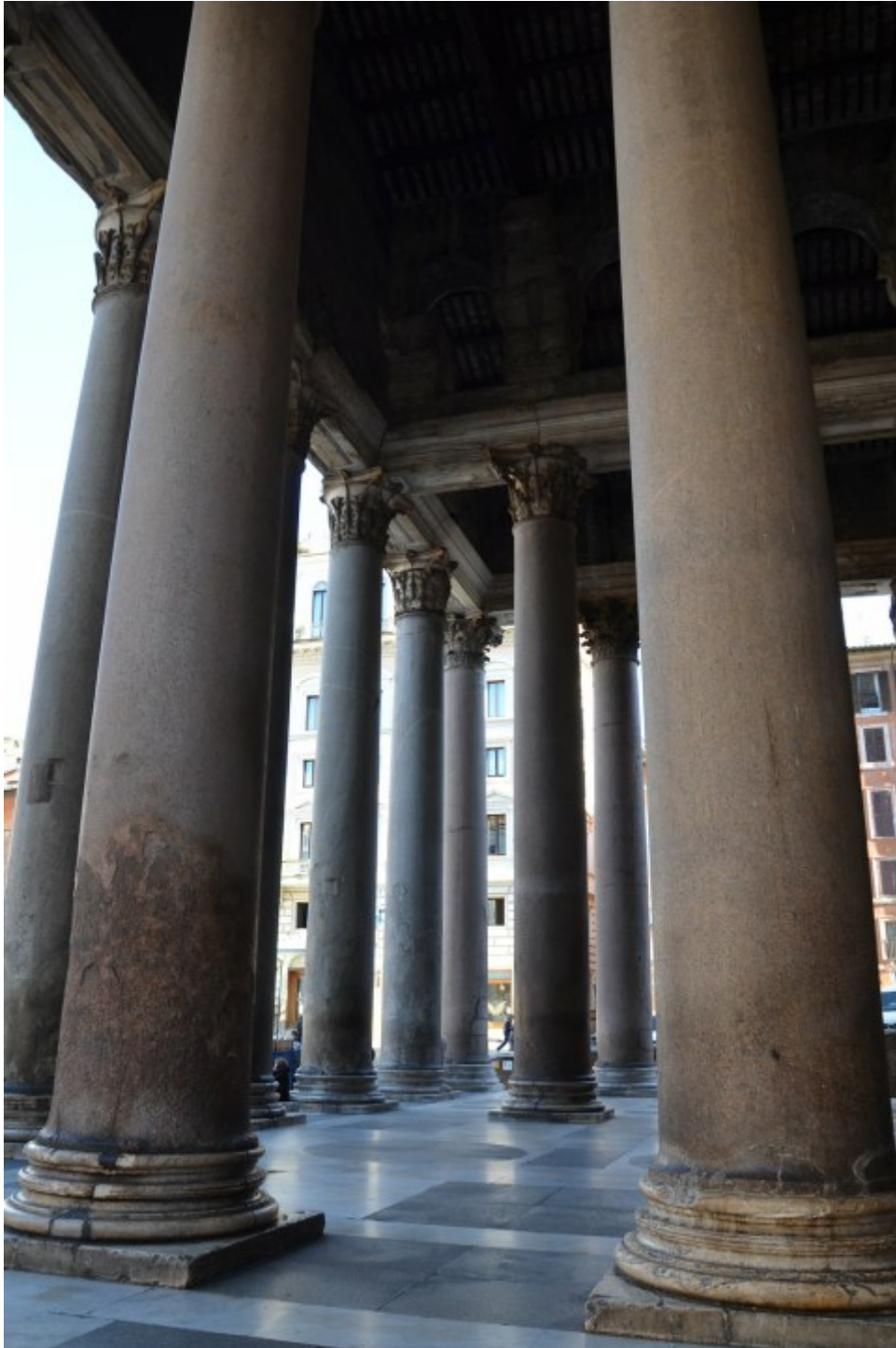
The Pantheon's porch was built in the traditional, Greek style of architecture, with columns holding up an entablature. Sixteen, monolithic columns form the monument's portico. The shafts are
